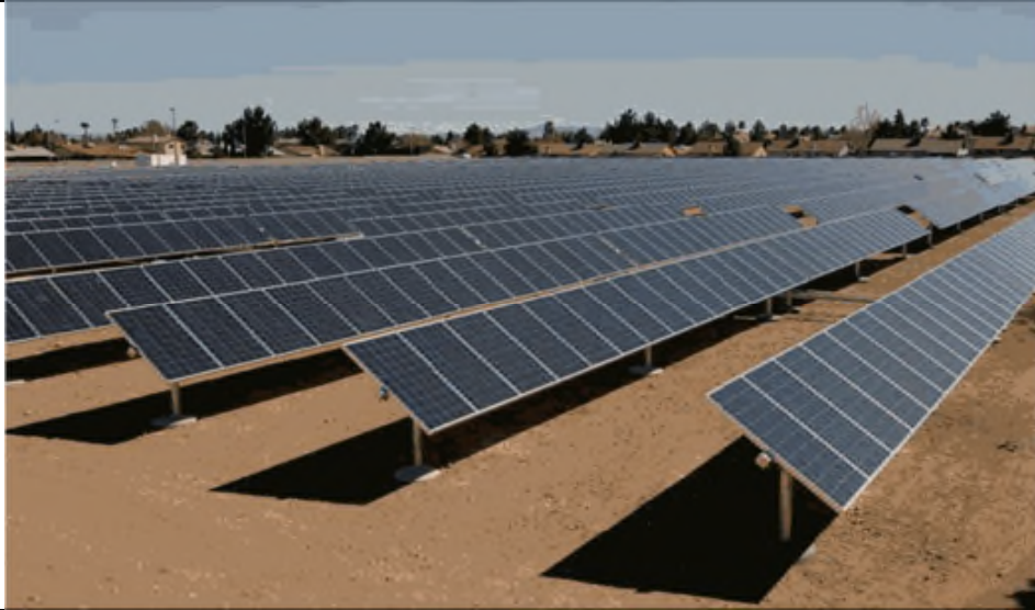
Plate 1. Fixed mounted PV system. Each unit is fixed in place orientated towards the sun's mid-day position
