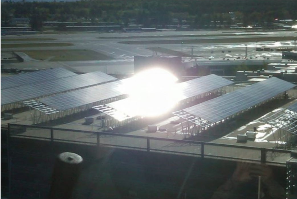
Plate 17 - Glare experienced in the Control Tower at Boston Regional Airport from a PV array
