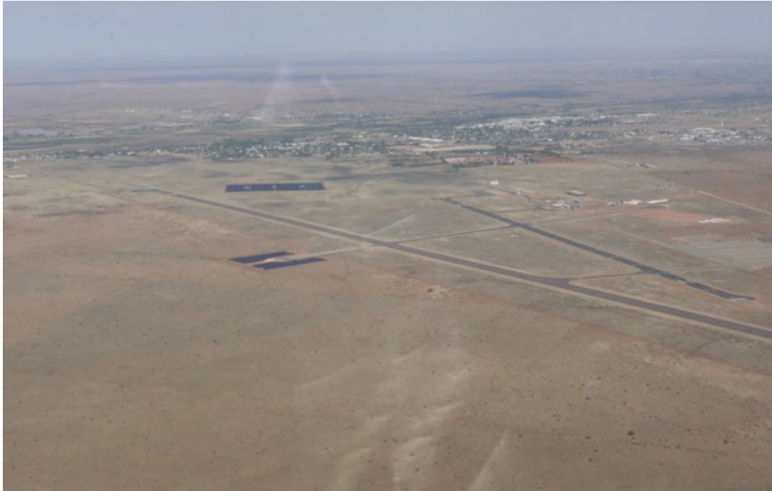
Plate 11 , Existing solar arrays at the Upington Airport as seen from the air
