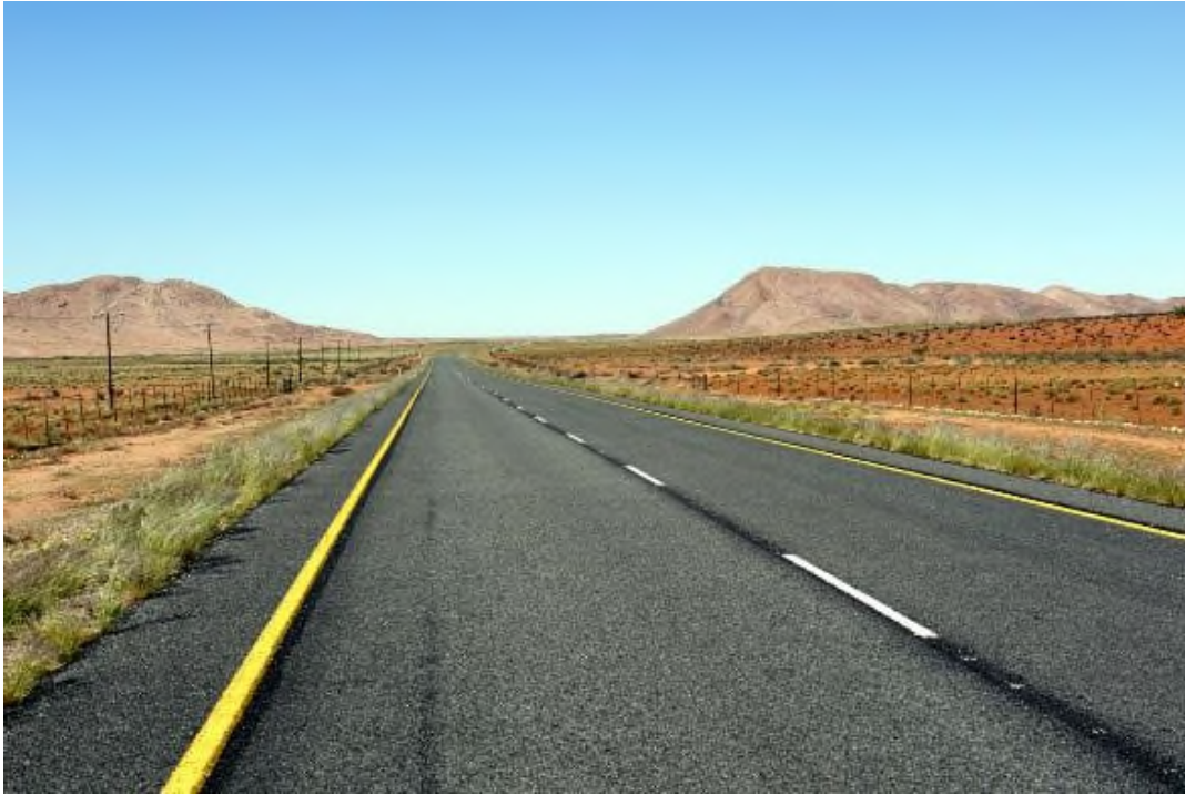
Plate 3, Inselbergs are often located close to and across the line of the N14. This creates the feeling for the traveller along the road of passing through a series of discrete landscape areas with each one being enclosed by the tall rocky landforms.
