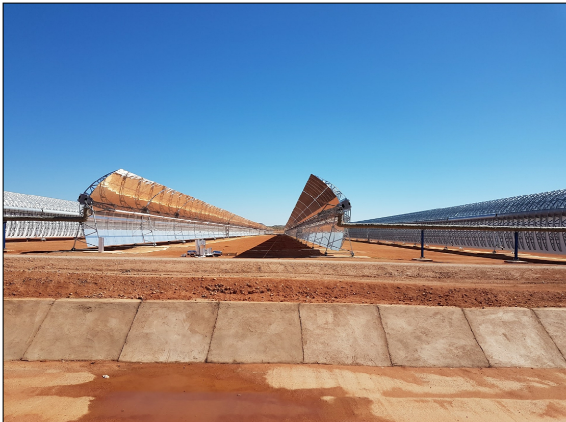
Figure 7: Solar Troughs at Ilanga 1 CSP. (Photo: Google Earth | Andrew Griffiths).
