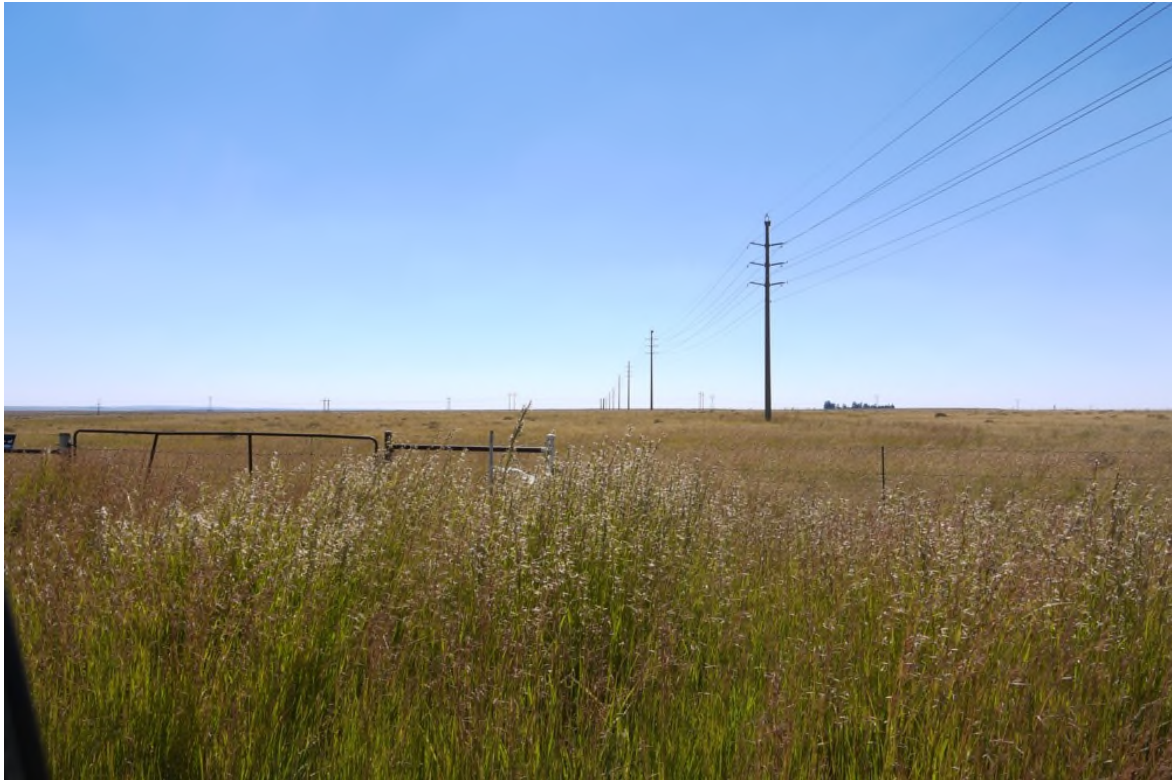
Plate 19, View of a 132kV overhead power line similar line to that proposed. Note pylons on the horizon (approx 2.5km distance) are just visible.
