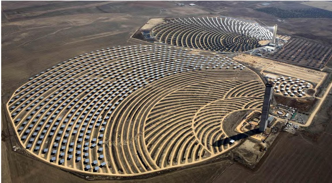
Plate 1, Existing Power Tower Projects in Sanlúcar la Mayor, near Seville, Spain. (photograph extracted from Desertec - UK web site, http://www.trec-uk.org.uk )
