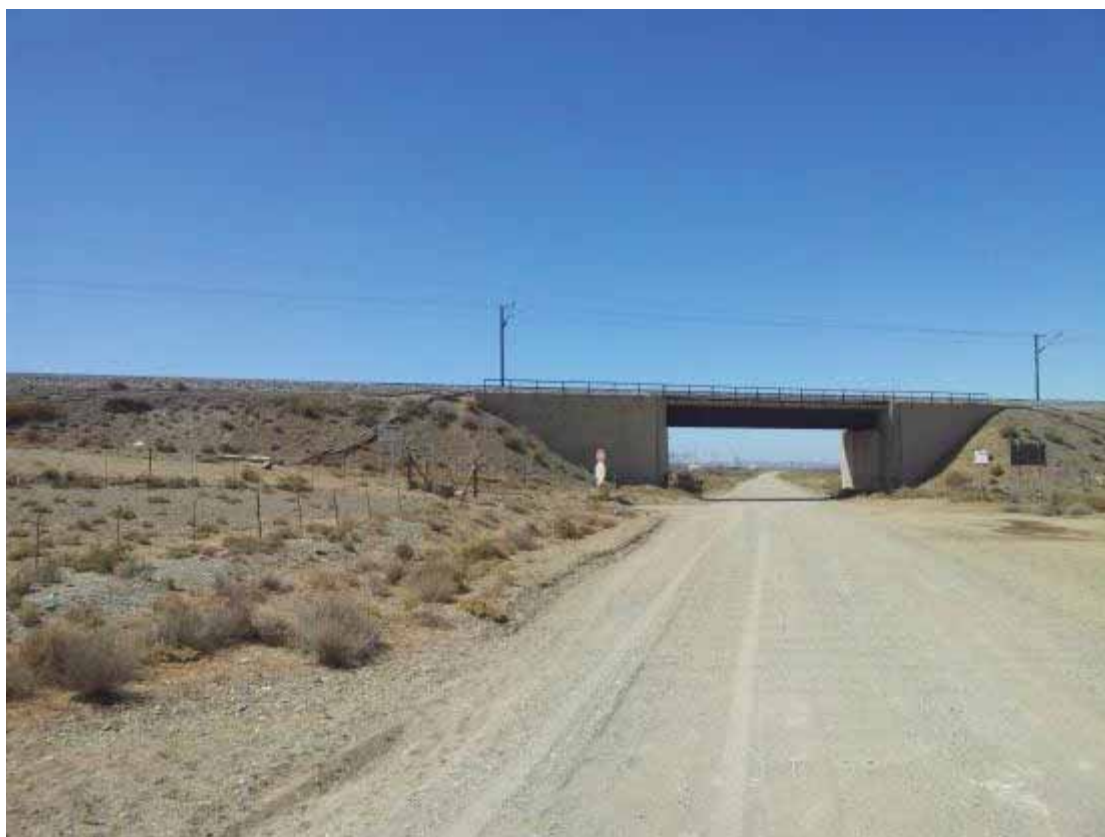
Photo 4.1 Railway Bridge Crossing
