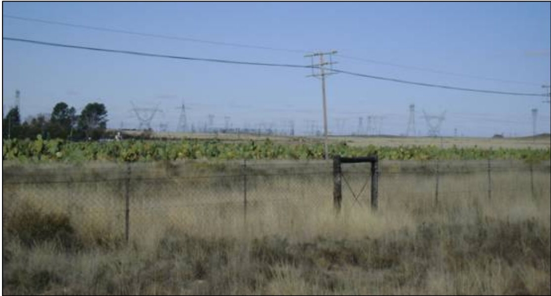
Figure 4: Power line infrastructure along the N10 south of De Aar.
