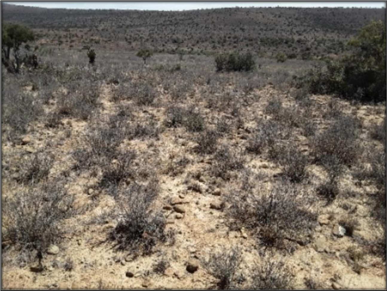
Figure 35: Hamlett Wind Energy Farm Collector substation area. Low vegetation and quaternary deposits. GPS -32.963889; 25.775556
