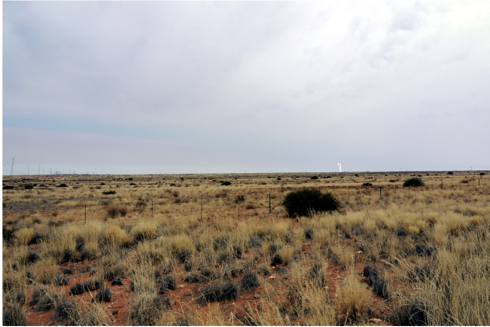
Plate 21, VP 2 – View looking to the south-west along an existing HV overhead power line from the Lutzputs Road. The existing Upington MTS is located to the left of plate 21. The existing Khi Solar One grid connection is just obvious on the horizon. The proposed power line alignment (to be developed within the grid connection corridor) will be viewed against this existing power line. The proposed alignment may be slightly more obvious as it will be closer to the road.
