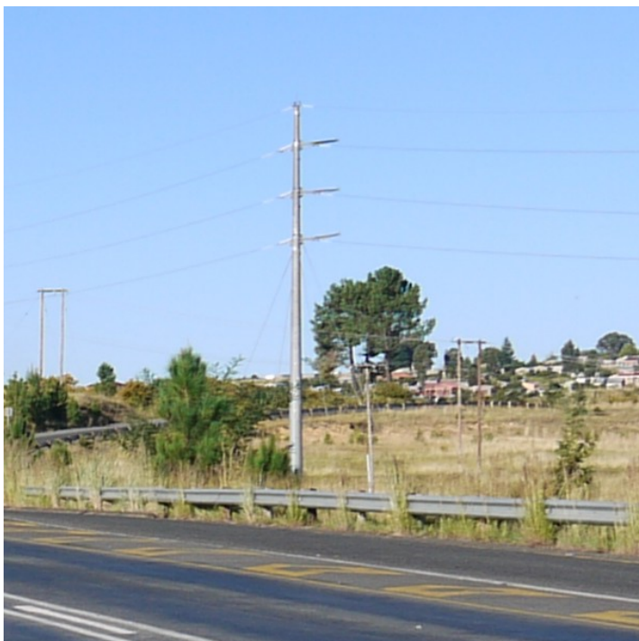
Plate 2 Eskom Monopole, 32m high.
