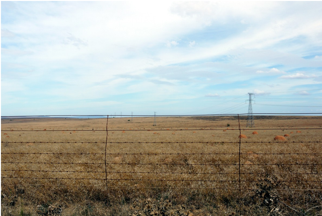
Plate 17 - A view along the line of an existing similar overhead power line with steel lattice towers
