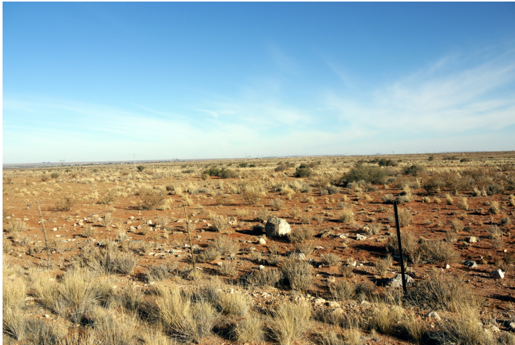
Plate 22, VP 3 – View looking to the south-west along two existing MV overhead power lines (left of picture) from the Lutzputs Road. The existing Khi Solar One grid connection is just obvious on the horizon. The proposed power line alignment, within the grid connection corridor, will be viewed against this existing power line. The proposed alignment may be slightly more obvious as it will be closer to the road.
