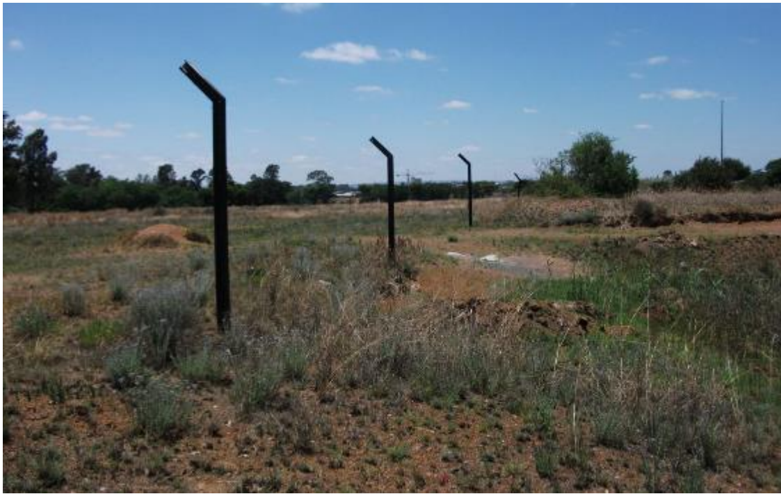
Figure 5: Fence posts on edge of dam
