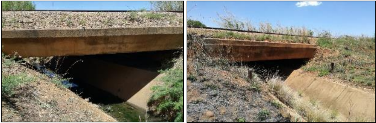
Figure 9: Two Bridges for Railway Lines
