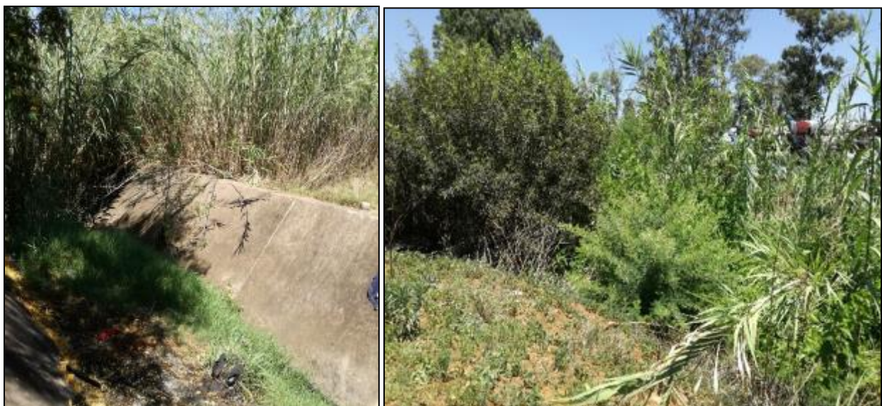
Figure 4: Overgrown Channel and Vegetation Restricting Access
