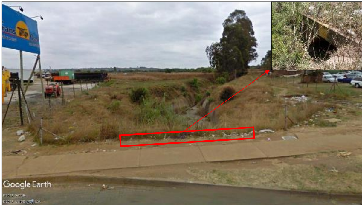
Figure 6: Triple barrel culvert by Stormvoel Road (Google Earth, 2010)
