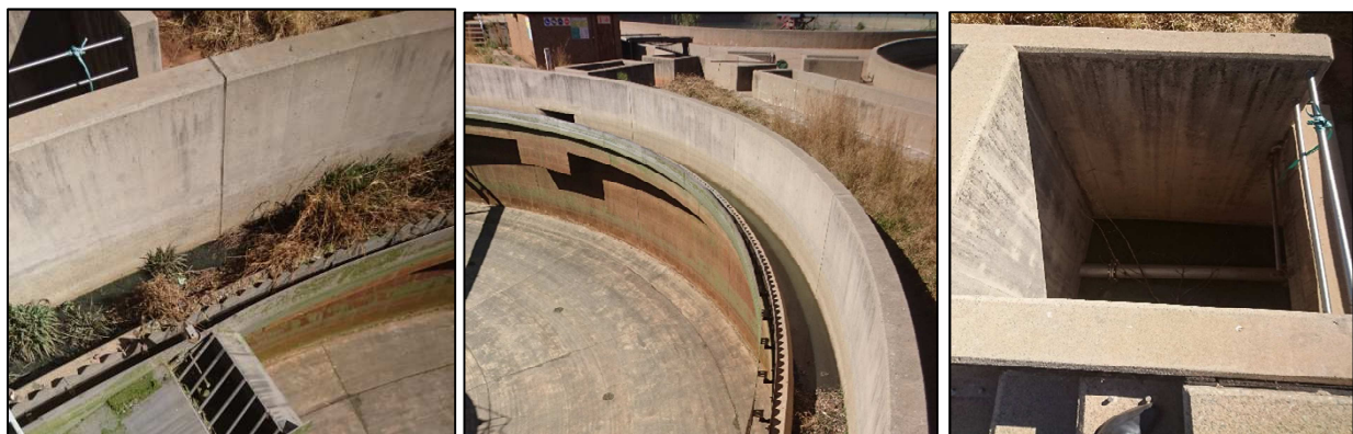
Figure 3: Concrete Walls of PST 5 and box
