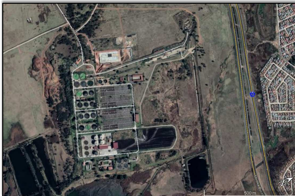
Figure 1: Aerial view of Bushkoppie WwTW
