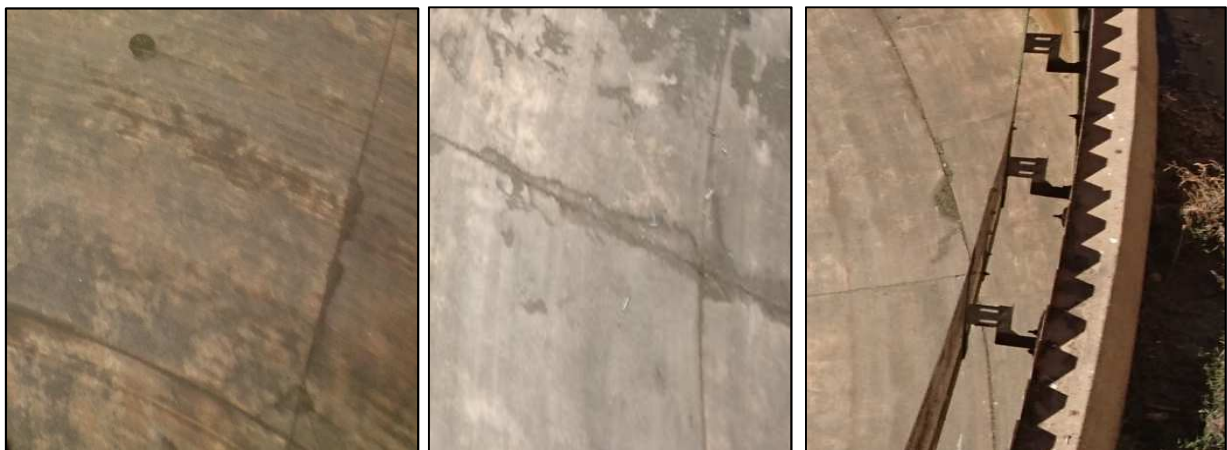
Figure 2: Floor joints in PST 5
