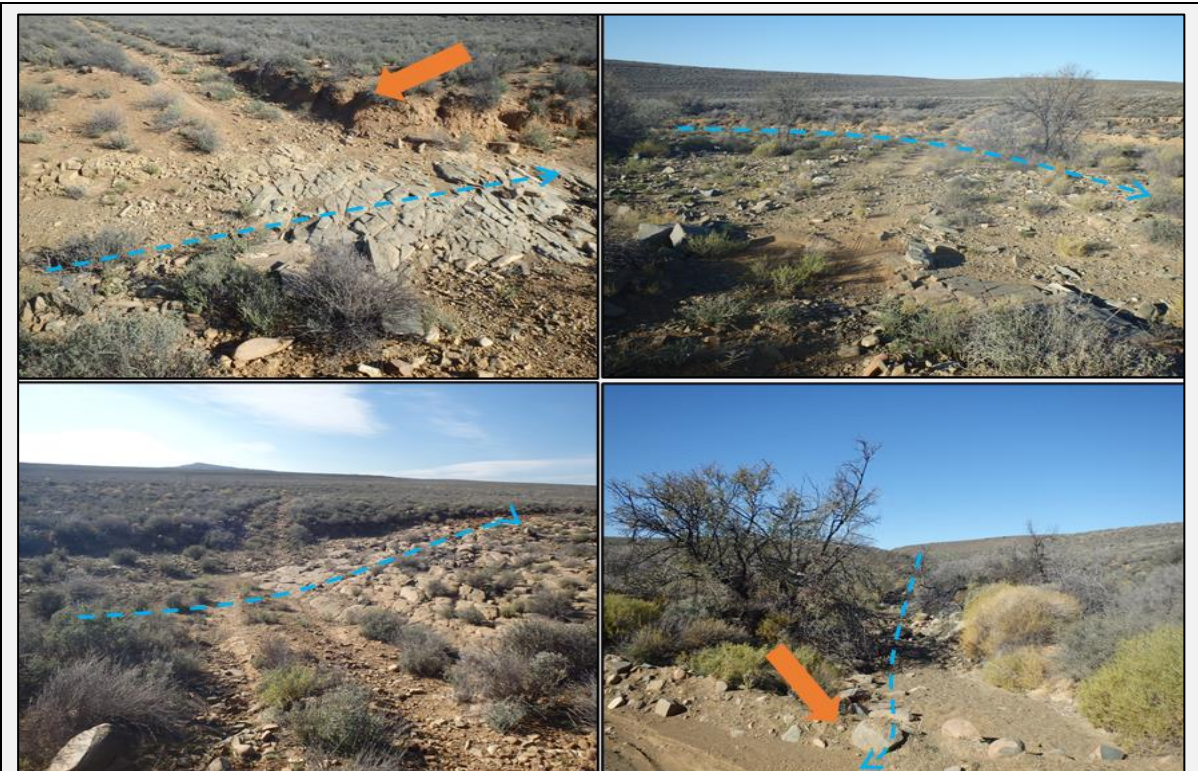
Figure 13: Various existing informal road crossings in and surrounding the proposed WEF development site through watercourses (blue dashed line), most of which are hosting a solid bed rock base. The orange arrow in the top left photograph depicts raised embankments, with minor erosion. Orange arrow in bottom right photograph depicts that despite not having any throughflow structures, the road crossing still allows for flow over the crossing.
