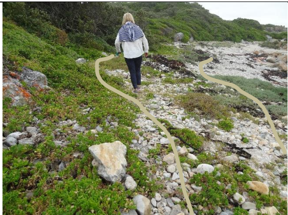
Figure 21: 5m 'construction zone' within which the ±1,2m wide path will be constructed, containing sparse hydrophytic vegetation
