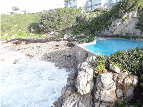
Figure 12: Present day appearance of pool at Bayview apartments
