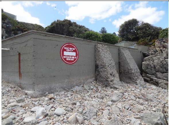
Figure 24: Pathway to follow edge of swimming pool at Bayview Apartments with no terrestrial vegetation occurring on rocky areas
