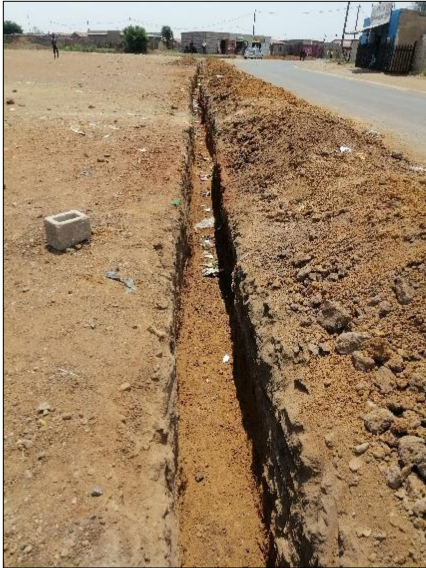
Photograph 2: Material Encountered in the existing trenches on site for the pipeline
