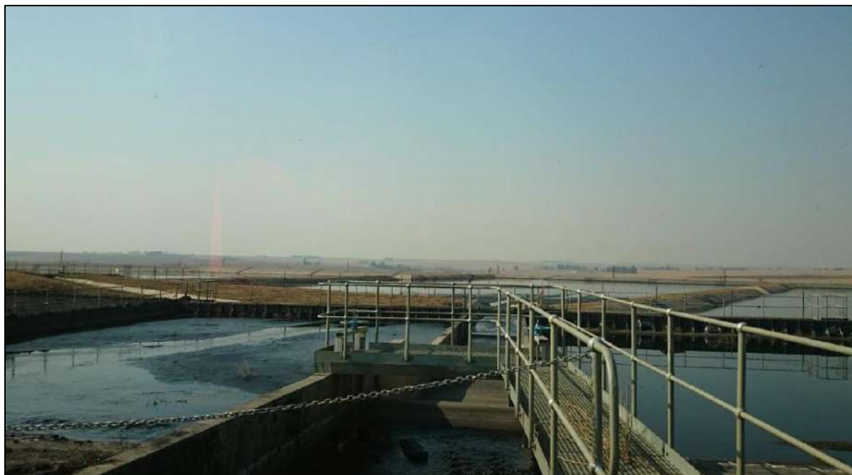
Figure 8.2: Side view of PCDs at DECM project site
