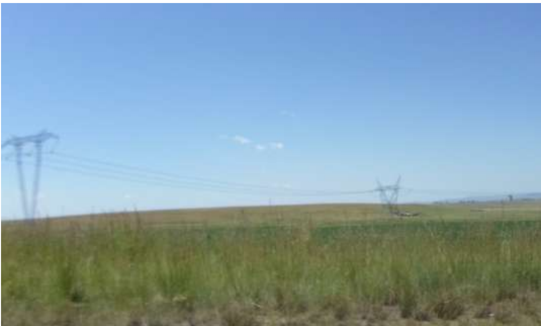
Figure 5: Adjacent farmland south east of Majuba Power Station (Power line and cultivated farmland on farm Witkoppies 3/81)
