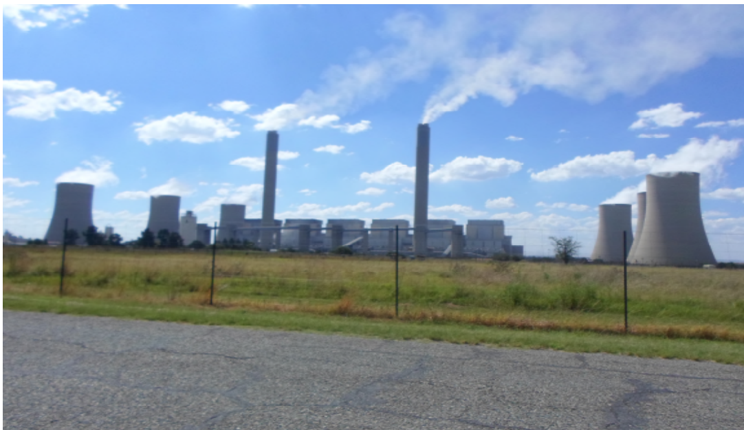
Figure 4: Lethabo Power Station & Alternative site 2 (Photo taken from the southern boundary of Farm 1814)
