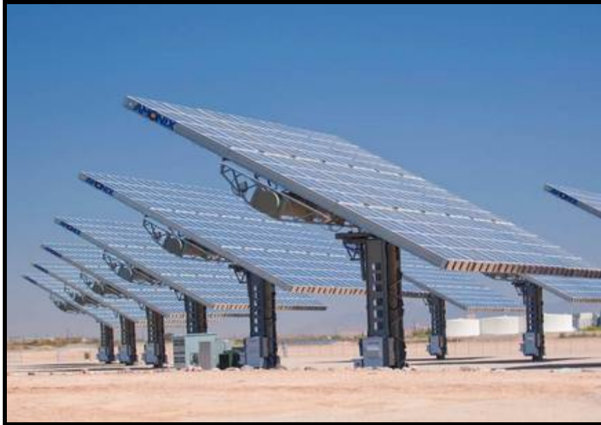
Figure 1.3: Illustration of a tracking solar energy facility (Courtesy of Amonix™)
