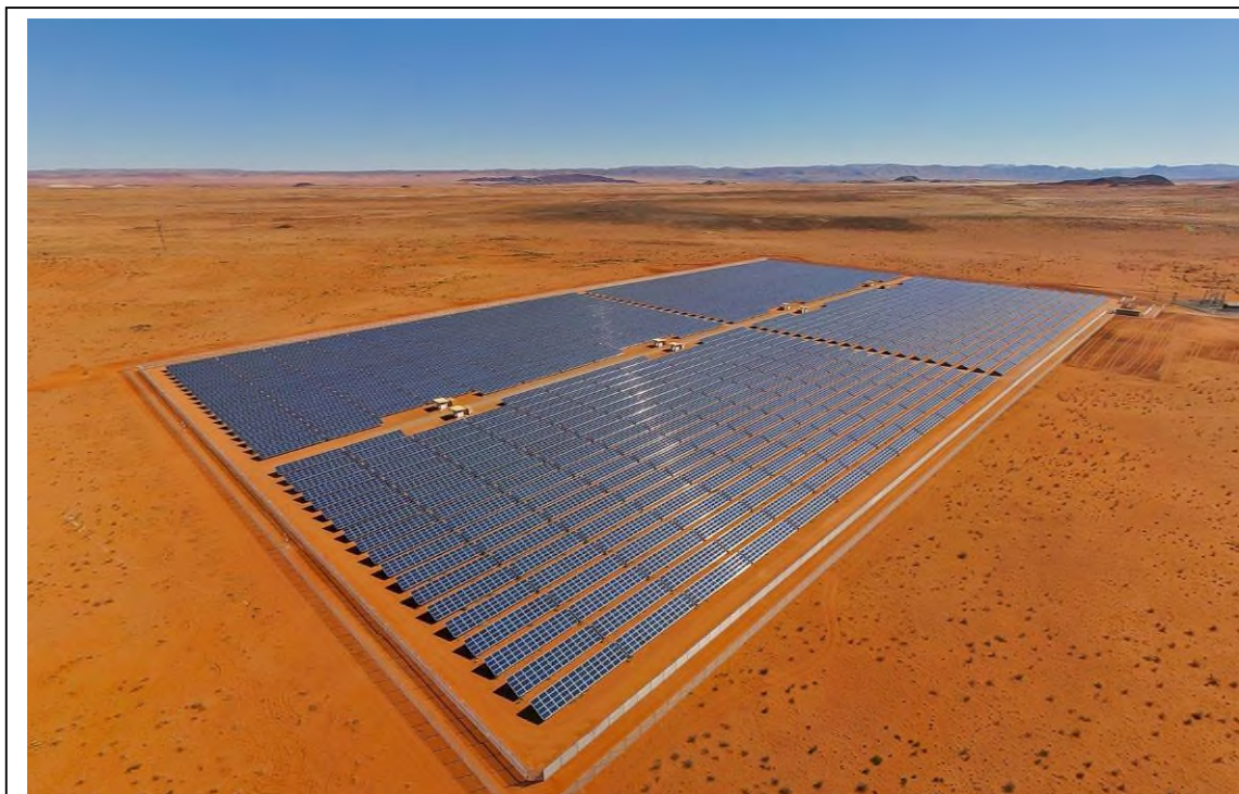
Figure 15: Konkoonsies Solar PV Plant on Portion 6 of Farm Konkoonsies 91 (Source: http://www.biothermenergy.com/blog/konkoonsies-solar-pv )
