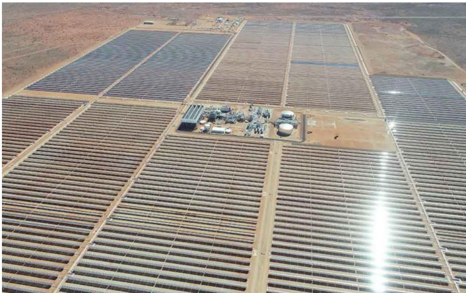
Figure 4.3: Operational Ilanga CSP 1 located in the north-western corner of Portion 3 of Lot 944 Karos Settlement (source: www.poweroilandgas.sener )
