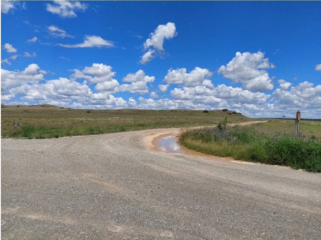
Photo 3-2: Proposed access to Riet Fountain Solar PV1
