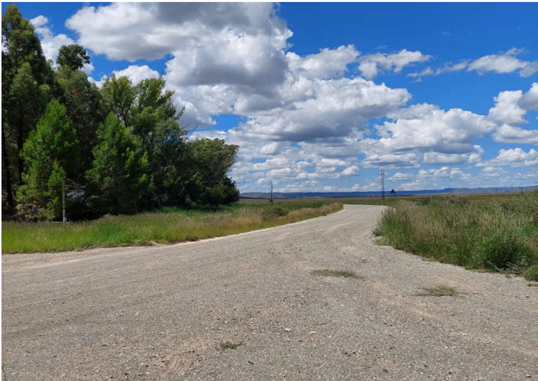
Photo 3-3: Insufficient shoulder sight distance to the East on proposed access to Riet Fountain Solar PV1
