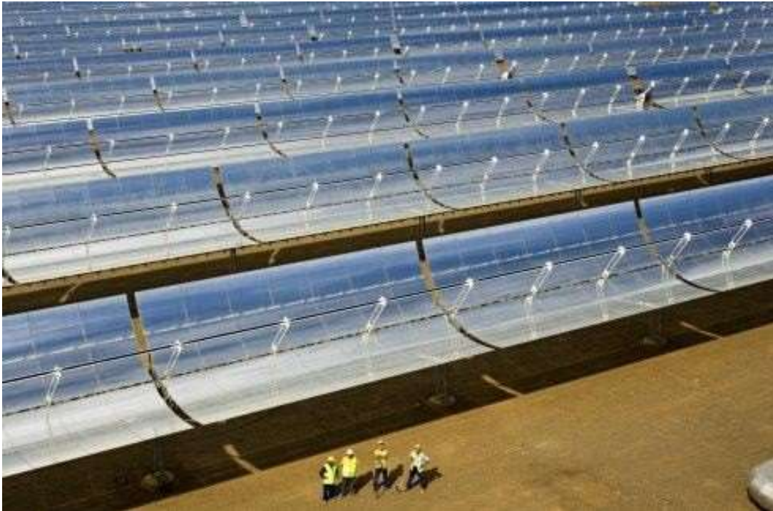
Plate 1, Existing Parabolic Trough Solar Field. (photograph extracted from solarhomes web site, http://www.jc-solarhomes.com )
