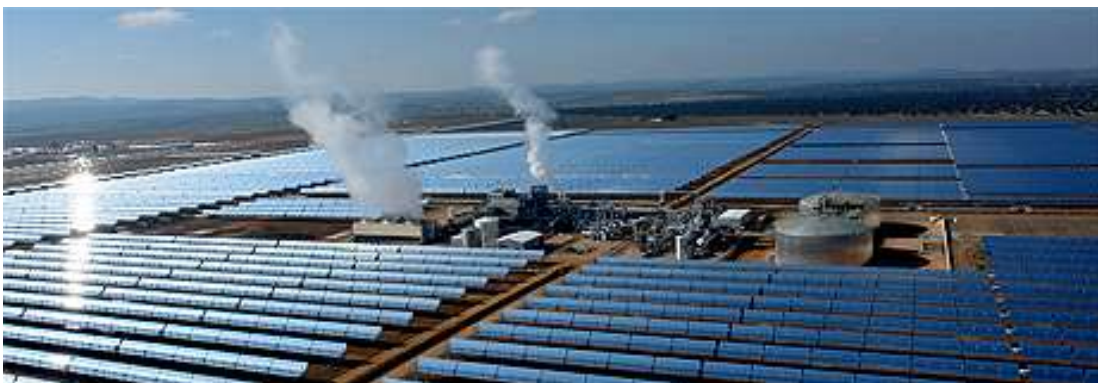
Plate 2, Existing 50MW Parabolic Trough CSP Plant in Torre de Miguel Sesmero, Badjoz, Spain. (photograph extracted from PennEnergy Web Site, http://www.pennenergy.com ). It should be noted that dry cooling technology is proposed for the projects under consideration in this report so there will be no steam visible from the cooling plant.
