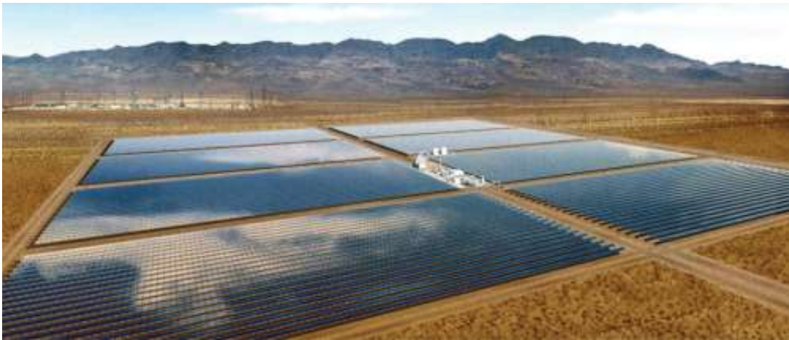
Plate 12, View of a parabolic trough CSP project from an elevated, close viewpoint (Renewable Energy Focus.com, http://www.renewableenergyfocus.com ). The structures visually combine to give the impression of an extensive industrial development.
