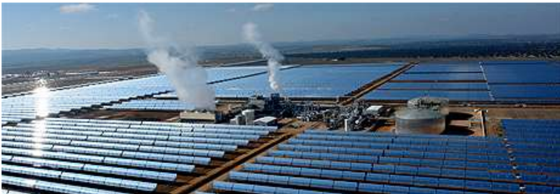
Plate 2, Existing 50MW Parabolic Trough CSP Plant in Torre de Miguel Sesmero, Badjoz, Spain. (photograph extracted from PennEnergy Web Site, http://www.pennenergy.com ). It should be noted that dry cooling technology is proposed for the projects under consideration in this report so there will be no steam visible from the cooling plant.
