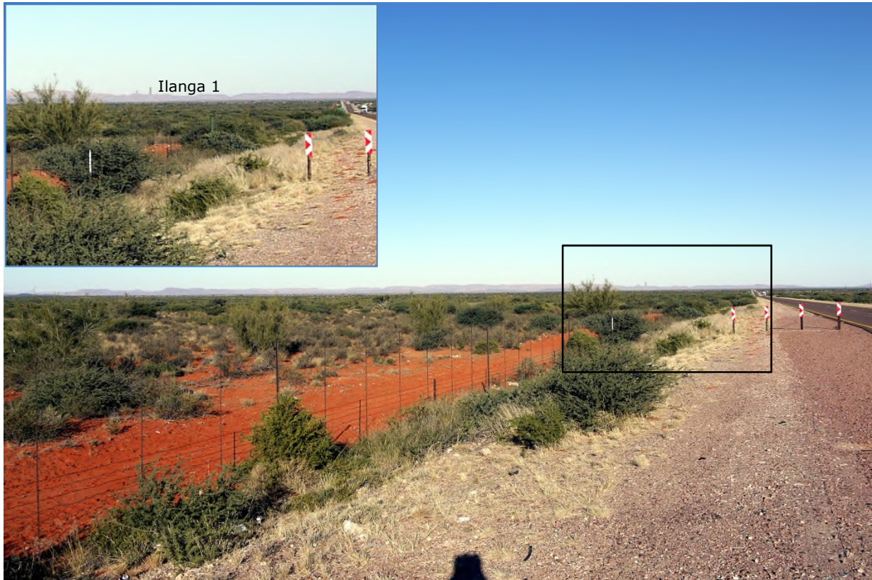
Figure 6, VP4 - View from the N14 close to FM Safaris approximately 34.0km from CSP7 Tower. In view from right to left are Ilanga 1 Tower (under construction) and CSP1 Tower (authorised). The ZTV analysis indicates that the CSP 7 and CSP8 Towers may be visible from this viewpoint however, the model does not indicate that they will be obvious. It may be that the very tops of the towers will be visible over the ridgeline. It should be noted that the receptor on the top of the towers will be on the opposite side of the structures. The diffuse reflection from these plates therefore should not make the towers more obvious.
