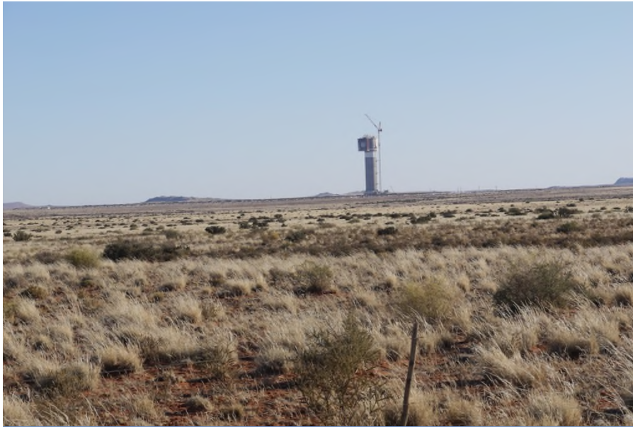
Plate 12, Existing Power Tower viewed from less than 5km.
