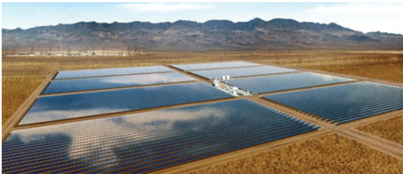
Plate 12, View of a parabolic trough CSP project from an elevated, close viewpoint (Renewable Energy Focus.com, http://www.renewableenergyfocus.com ). The structures visually combine to give the impression of an extensive industrial development.
