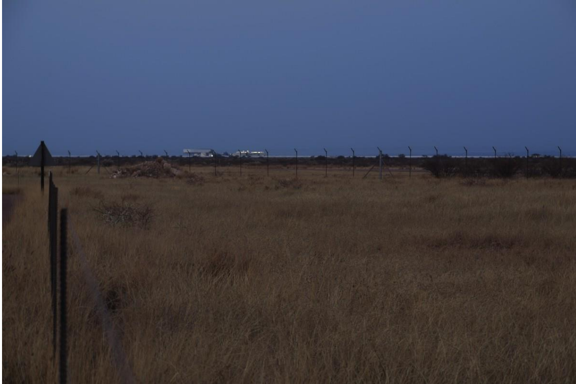
Plate 9, View of Kalahari Solar Power Project at night from the Kathu Airport
