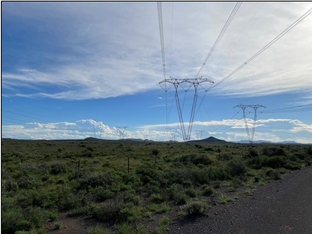
Figure 10: Existing power lines crossing the Hutchinson secondary road (looking to the south-west).
