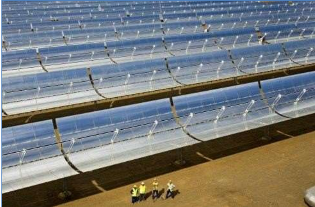
Plate 1. Example of existing Parabolic Trough Solar Field. (photograph extracted from solarhomes web site, http://www.jc-solarhomes.com )
