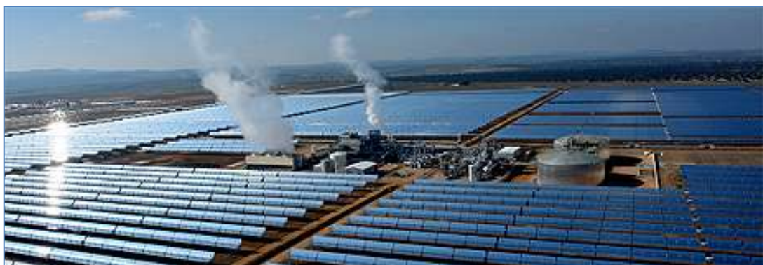
Plate 2. Example of existing 50MW Parabolic Trough CSP Plant in Torre de Miguel Sesmero, Badjoz, Spain. (photograph extracted from PennEnergy Web Site, http://www.pennenergy.com ). It should be noted that dry cooling technology is proposed for the project under consideration in this report so there will be no steam visible from the cooling plant.
