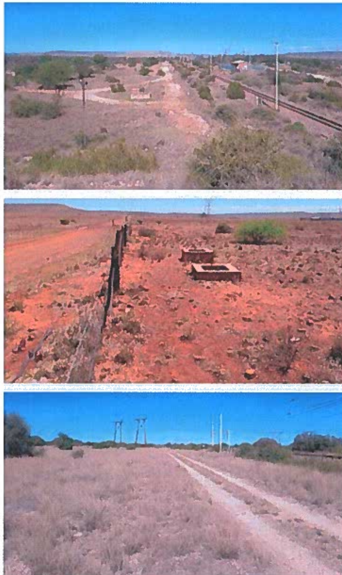
Figure 3: Views along the existing pipeline servitude
