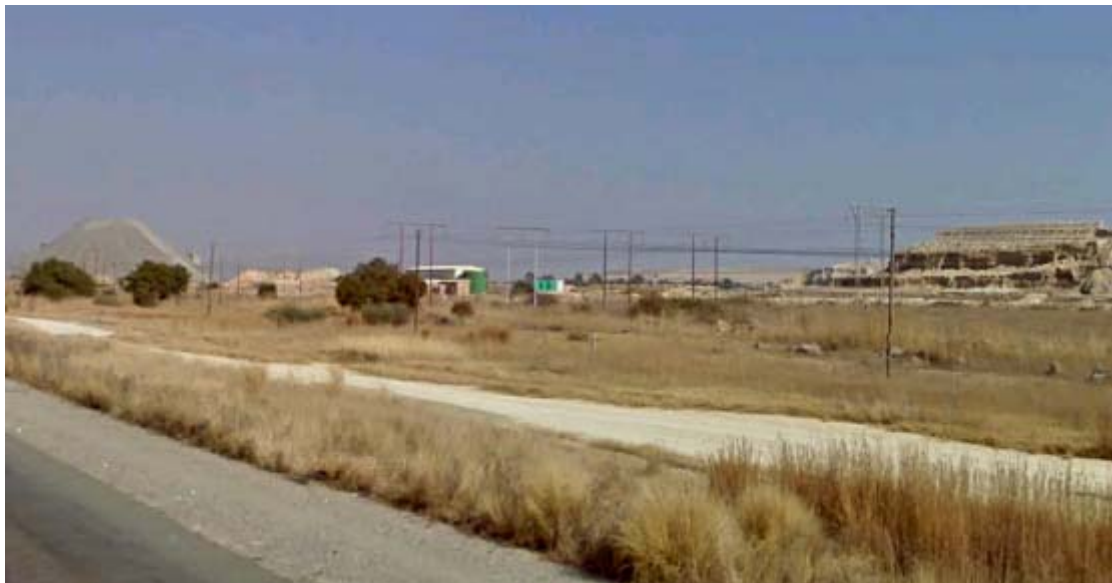
Figure 2: View of power lines between the R502 and an old slimes dam.
