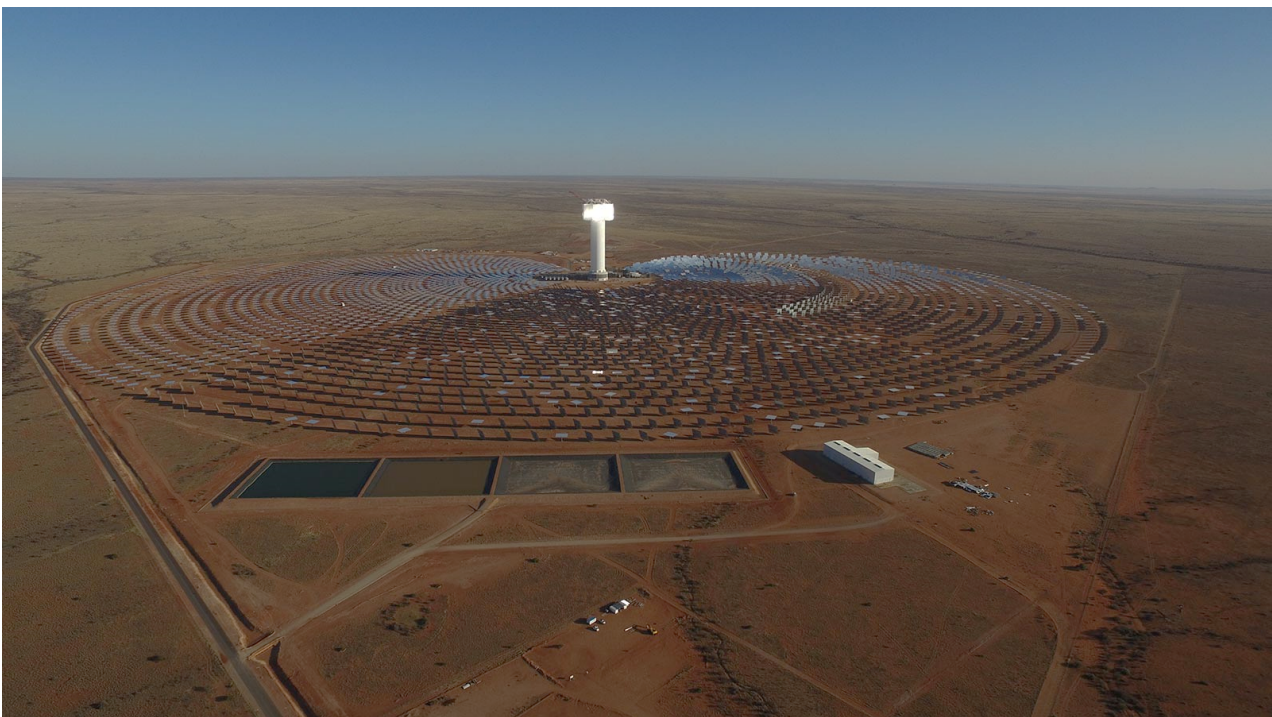
Figure 4.3: Operational Khi Solar One located (source: www.energy.org.za )
