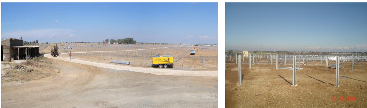
Figure 11: Illustration of a typical site after preparation
