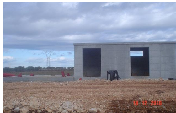
Figure 9: Foundation of a typical onsite building
