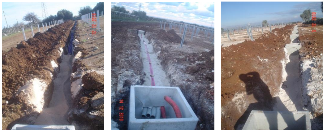
Figure 8: Cable trenches
