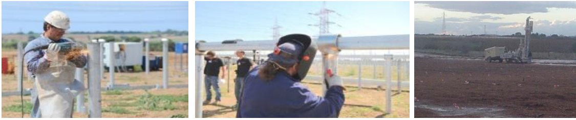
Figure 12: Onsite construction of the PV arrays
