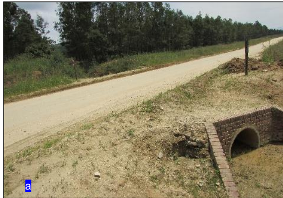
(a): Image showing existing structure at RC1 and P303 road. Note sedimentation of pipe; (b): Image showing upstream characteristics of the existing P303 structure (c): Additional image showing downstream of RC1.
