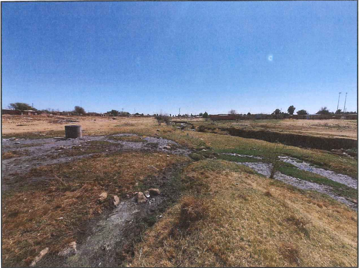
Figure 6: Overflowing Manholes near watercourse entering Pumping Station B
