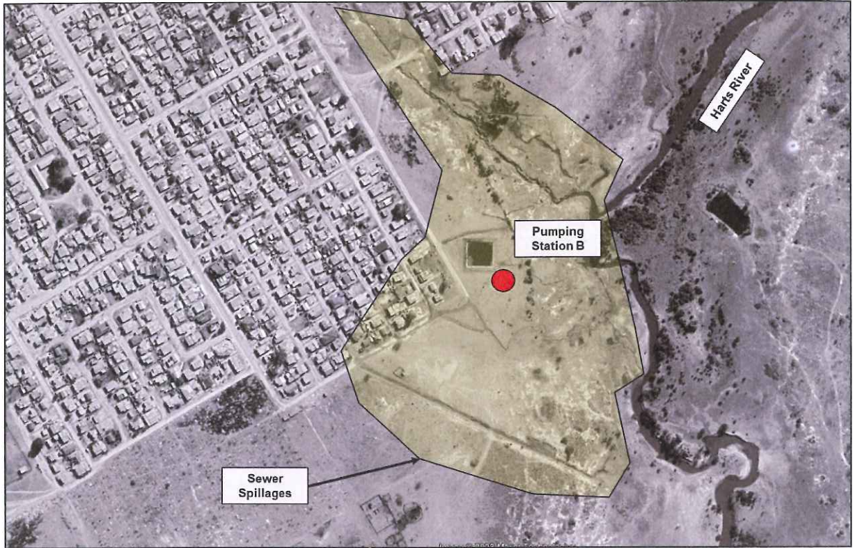
Figure 5: Aerial View of Sewer Spillages at Pumping Station B
