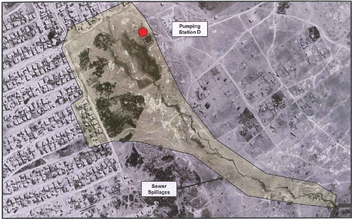
Figure 7: Aerial View of Sewer Spillages at Pumping Station D
