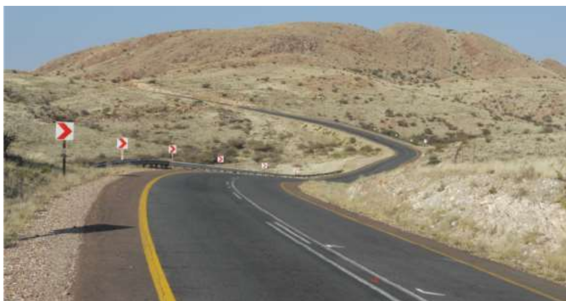
Figure 2: N10, kilometre chainage 87.2
