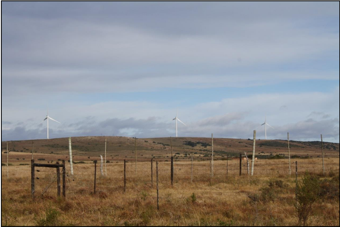
Figure 4: Wind turbines at the Waainek WEF.
