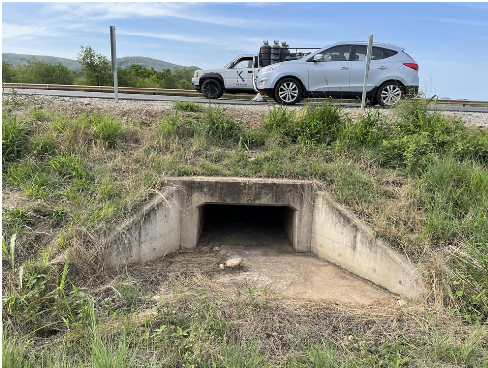
Photo 6: Smaller stormwater culvert under N4 in approximate middle of study site
