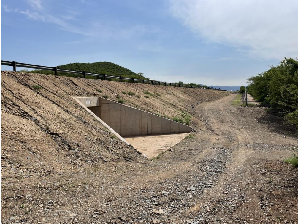
Photo 5: Stormwater culvert under N4 in area of southeast corner of site
