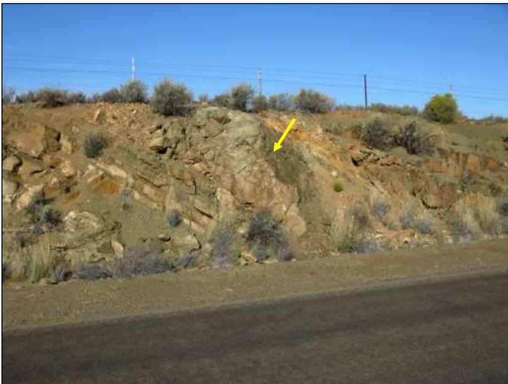
Figure 44. Disturbed bedding either side of a fault zone marked by massive fault breccia (arrow), R354 road cutting, Roode Wal 187 (Loc. 028).
