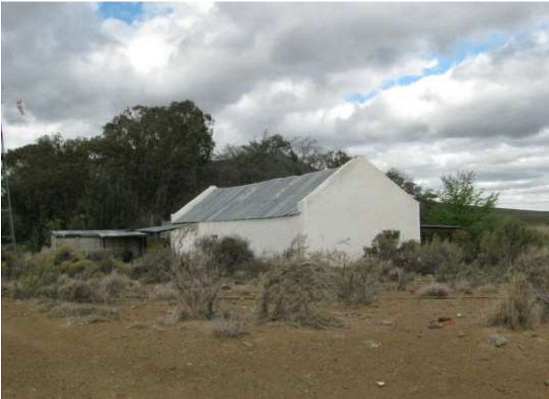
Figure 7. Existing structure, Ekkraal.
