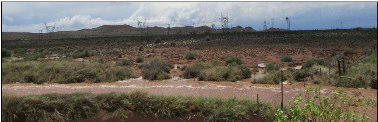
Photograph 3.3: Portion of Gamma substation located just to the north of the R63
