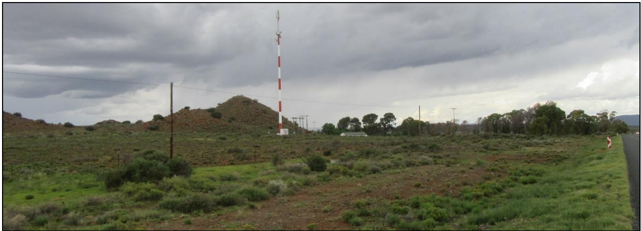
Photograph 3.5: Cell phone relay tower along the N1 on Vogelstruisfontein Farm
