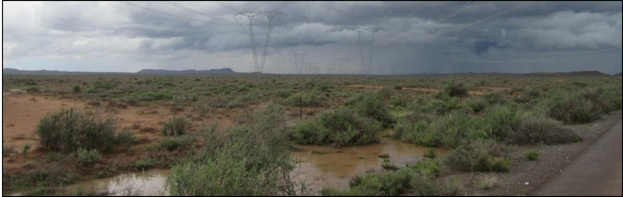
Photograph 3.4: Four (2 X 400 kV and 2 X 765 kV) Tx lines traversing the Hutchinson Road within a 350 m corridor on Annexe Rondawel
