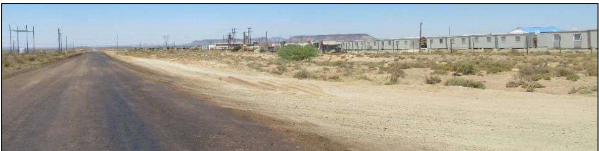
Photograph 3: The Granaatboskolk gravel road seen during the construction of Khobab WEF, December 2016.
