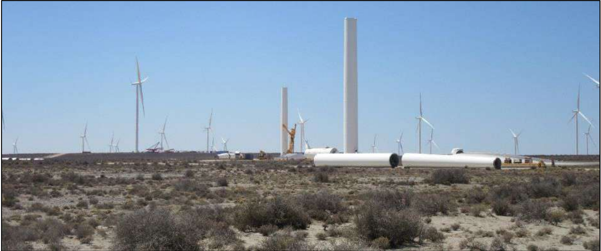
Photograph 1: Loeriesfontein WEF under construction, seen from, the Granaatboskolk gravel road, December 2016.
