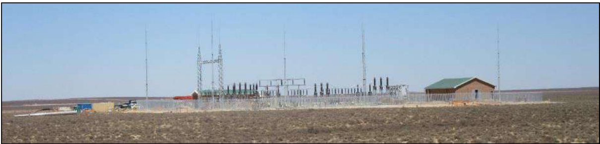
Photograph 2: Khobab WEF substation under construction, seen from, the Granaatboskolk gravel road, December 2016.
