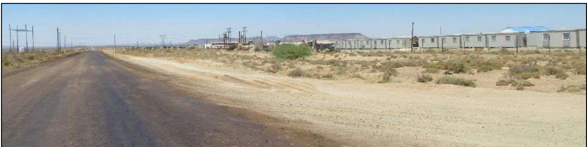
Photograph 3: The Granaatboskolk gravel road seen during the construction of Khobab WEF, December 2016.
