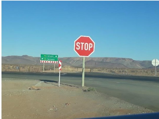
Photograph 5.1: Access off N14
