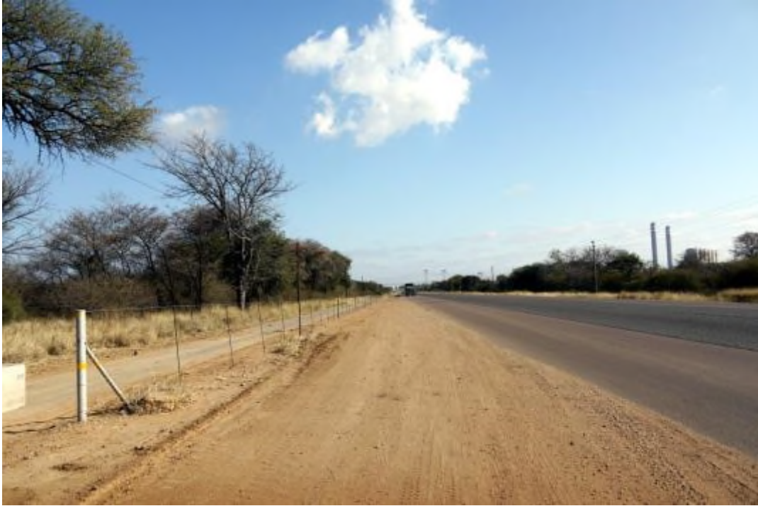
Plate 6, View from areas close to the Industrial ZTV from which partial views of the proposed development, may be visible
