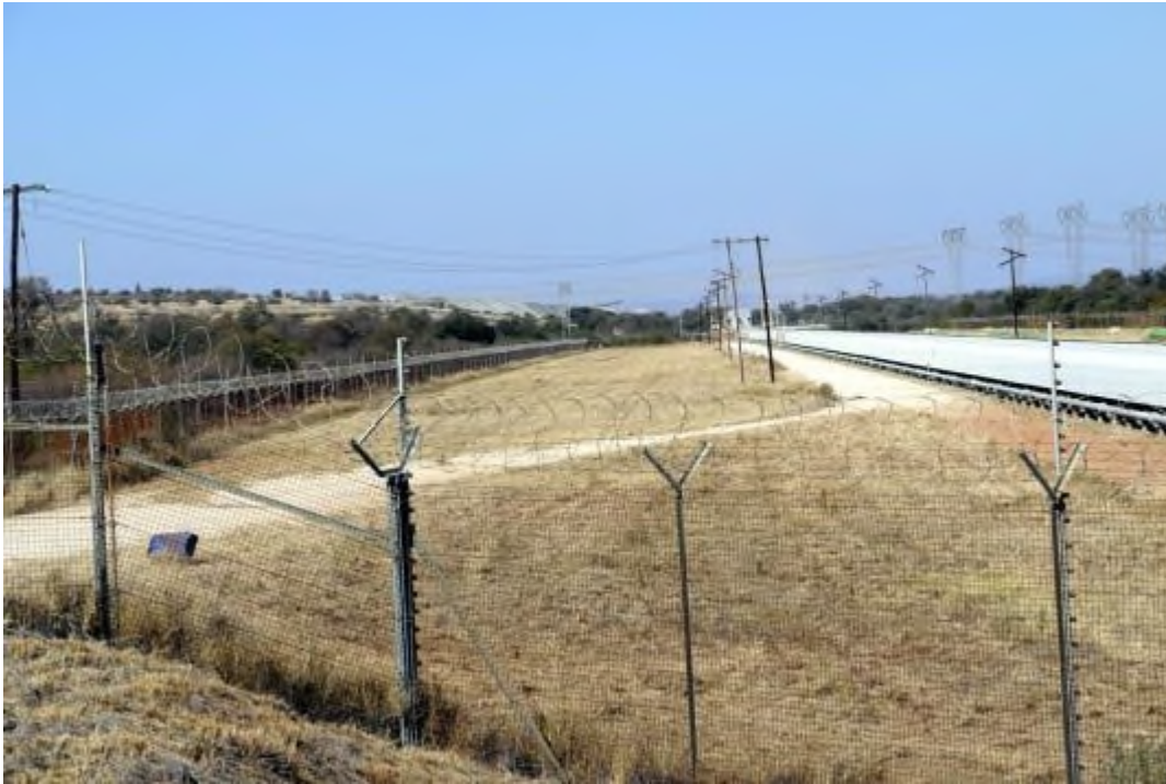
Plate 2, Conveyor delivering PFA to the ashing Facility associated with the Matimba Power Station. Note the elevated conveyor approximately centre of image that is dumping ash on the dump as well as the covered conveyor to prevent wind blow of ash. The ashing facility will gradually grow during the life of the power station. Vegetation that has established on the ash dump helps to disguise the fact that it is a waste dump.
