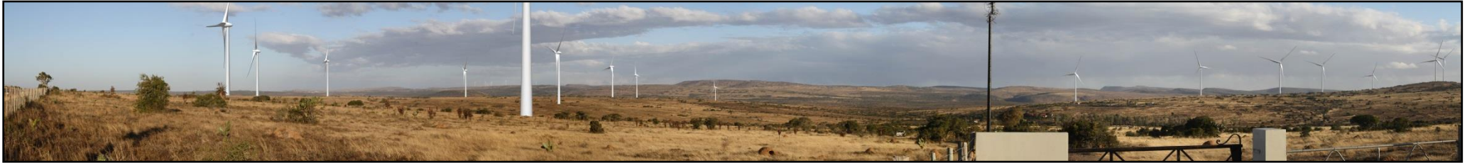
7.2. Viewpoint 1: after construction (Figure 13: Photo simulation 1 - after). The closest wind turbine is 400m from this point.
