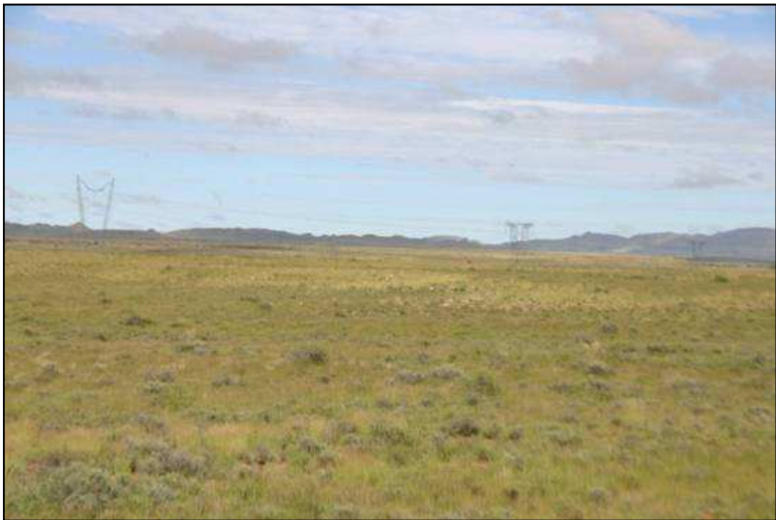
Figure 6: Existing overhead power line infrastructure to the south-east of the proposed site.
