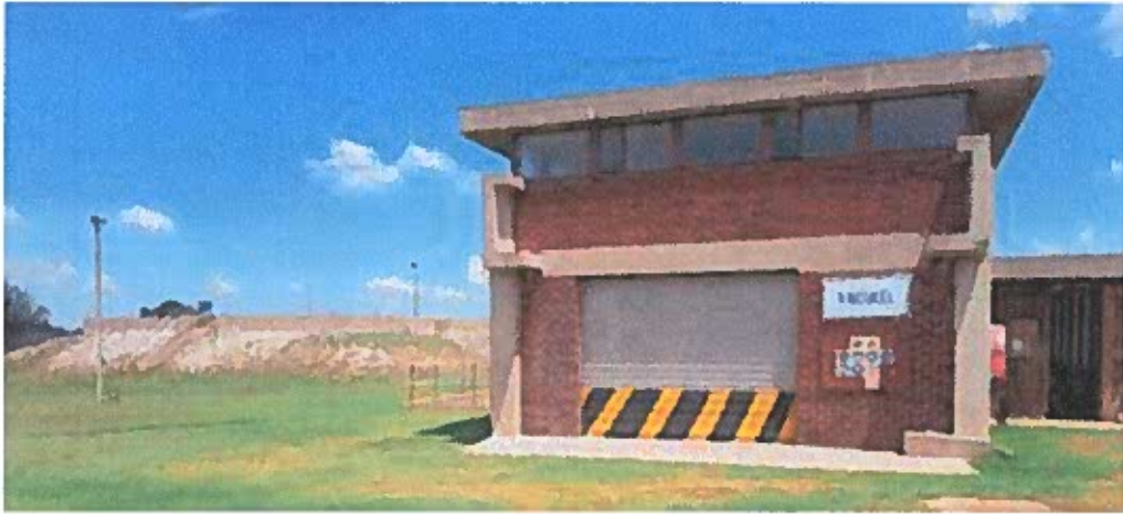
Figure 4: Kneukel Pump Station and Sump
