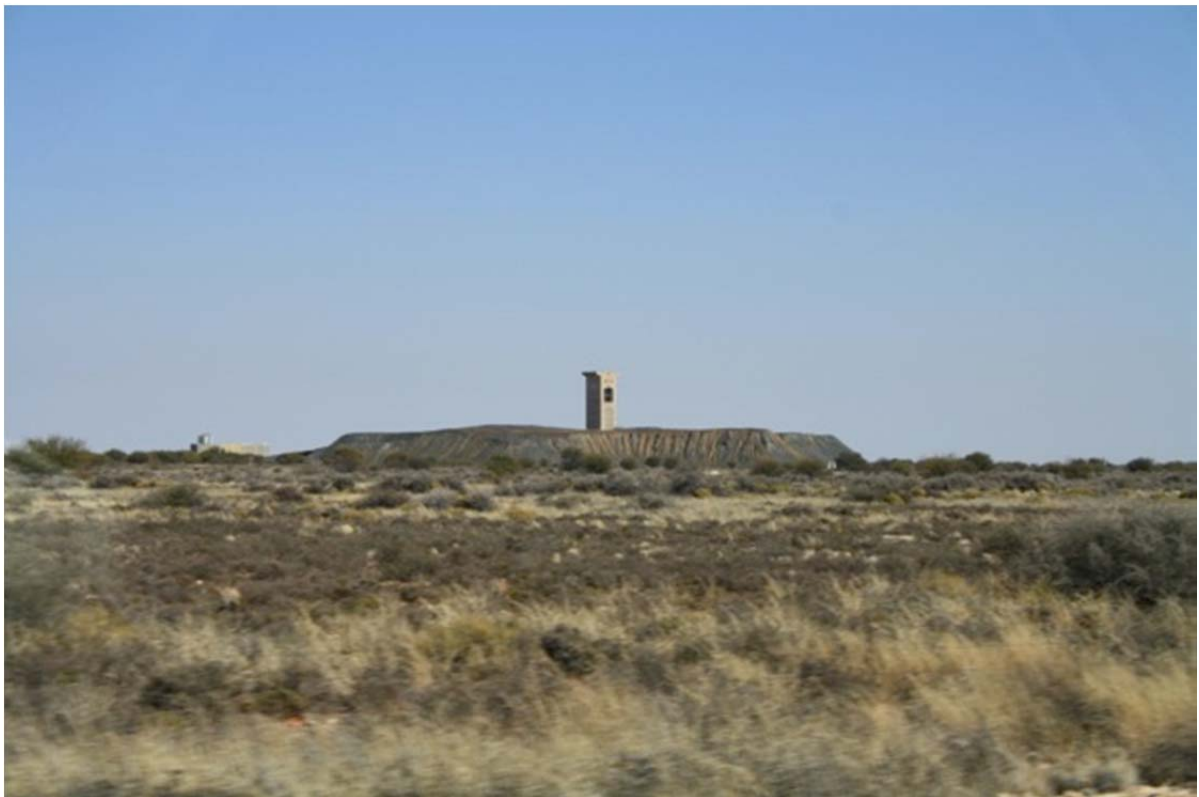
Figure 5: Infrastructure associated with the Copperton Mine.
