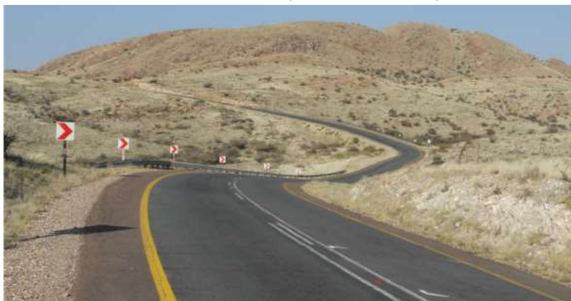
Figure 2: N10, kilometre chainage 87.2
