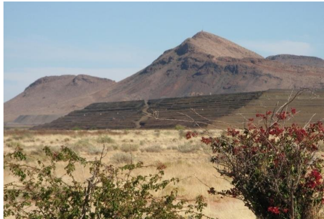
Plate vi: Mining: Black Mountain tailings dam
