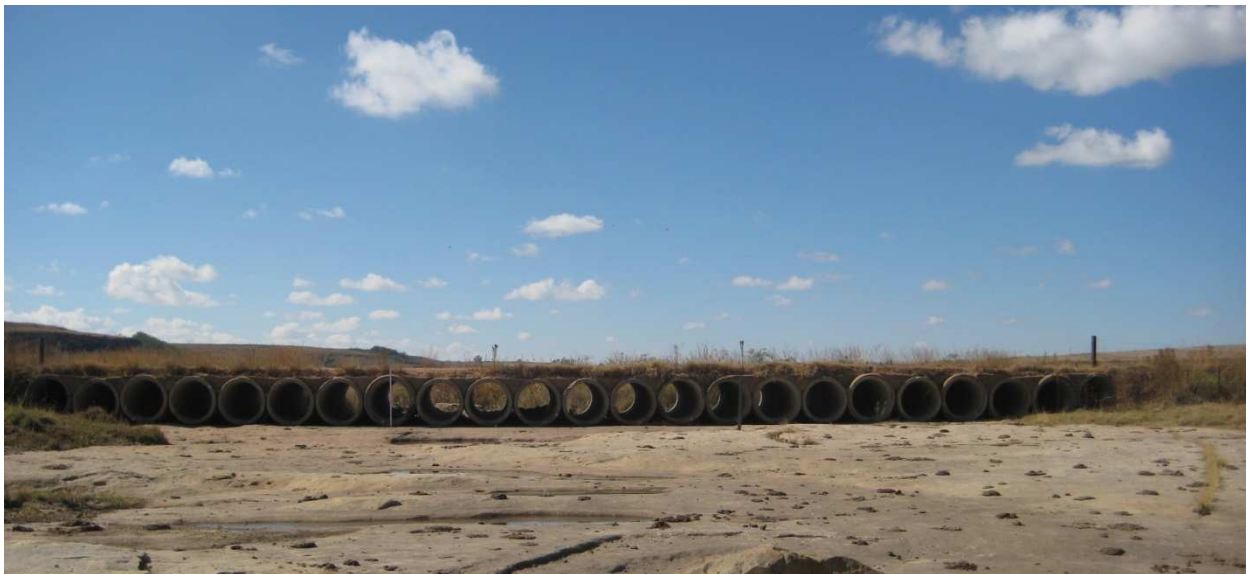
FIGURE 5-3: RIVER CROSSING OVER STEENKOOLSPRUIT MAIN CHANNEL NORTH-EAST OF SHAFT COMPLEX - FACING UPSTREAM (EAST)
