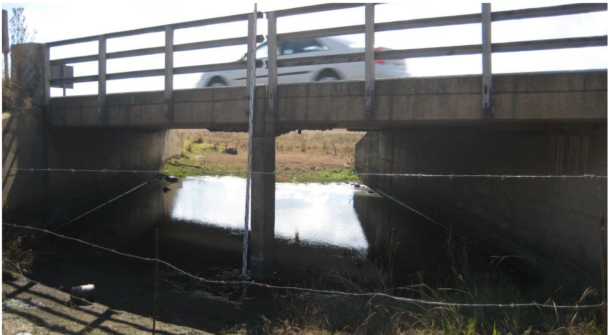
FIGURE 5-5: BRIDGE OVER STEENKOOLSPRUIT TRIBUTARY 2 - FACING DOWNSTREAM (NORTH)
