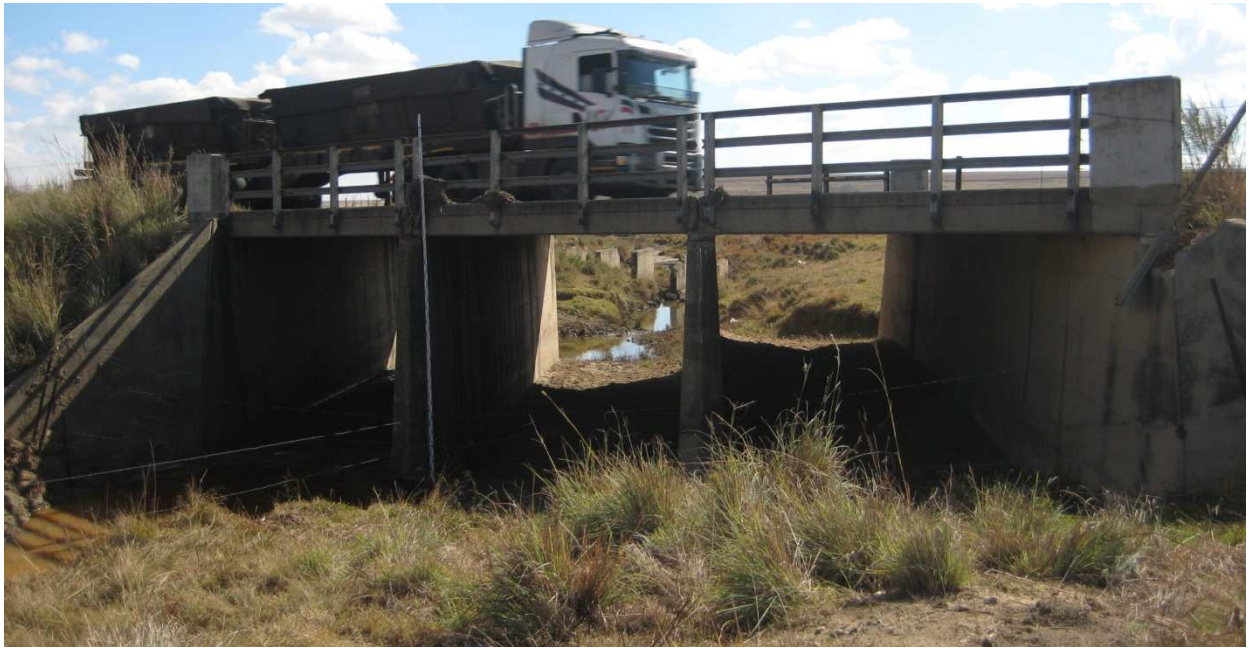
FIGURE 5-2: BRIDGE OVER STEENKOOLSPRUIT TRIBUTARY 1 - FACING DOWNSTREAM (NORTH)
