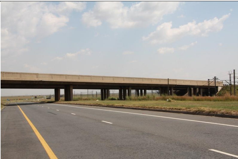
Bridge on N12 – east side of project
